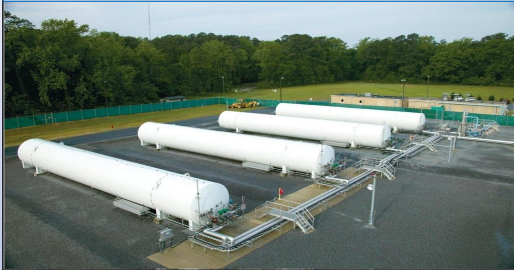
LNG Storage and Control Building
