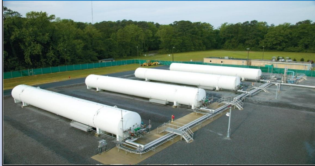
LNG Storage and Control Building
